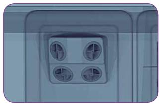
**Image 2.** Specially designed vents to provide complete 3-D surface coverage during HPV bio-decontamination
